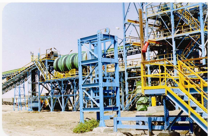
● Redeyef washing plant
